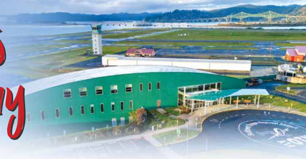
Southwest Oregon Regional Airport
